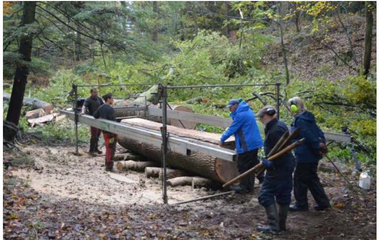
Sawing in progress. Photo: Nigel Gutteridge
